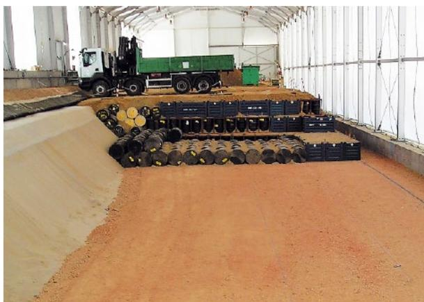
Figure 2. General view of VLLW trench at El Cabril disposal facility [15]
